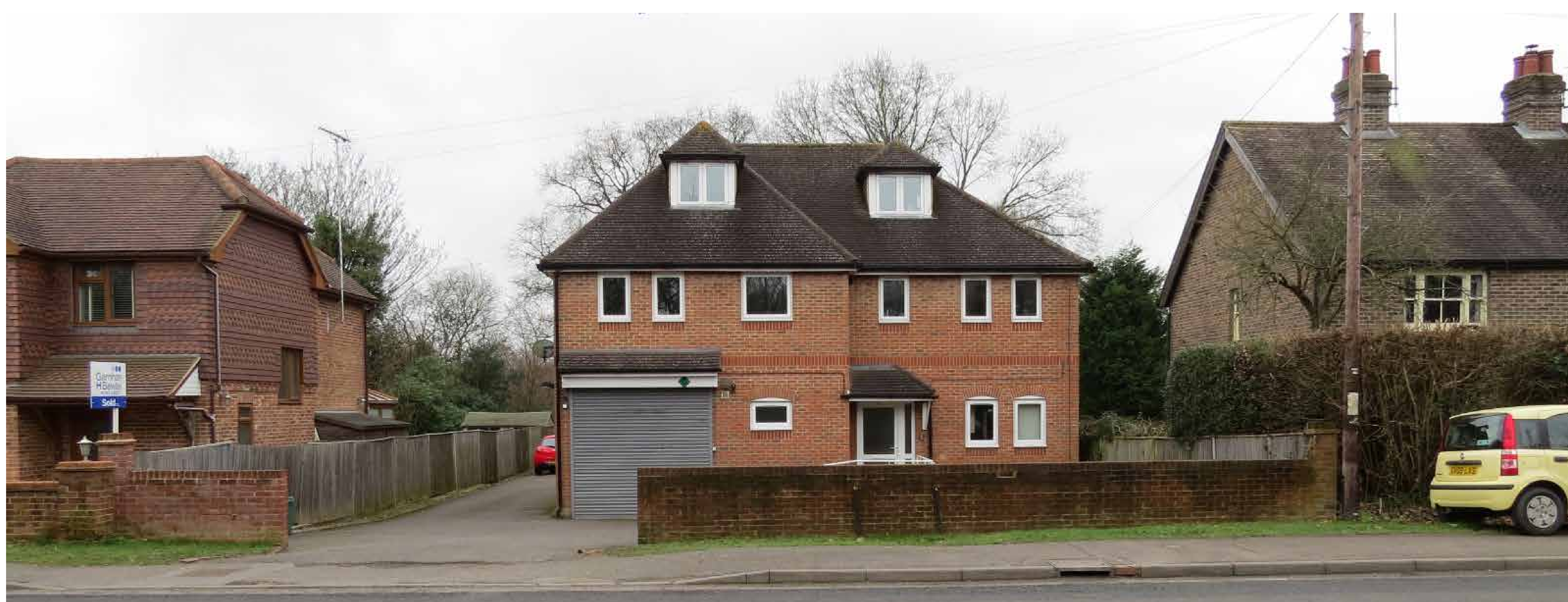
FORMER ST. JOHN AMBULANCE BUILDING TO BE DEMOLISHED TO PROVIDE ACCESS
